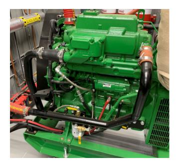
2. John Deere 6068AFM - Remove coolant tank and other accessories that are
