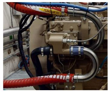
3. John Deere 6090AFM - Remove coolant expansion tank and other accessories that are not required. Manifold vent lines into a single air vent/pre-heat connection near the front. See photograph for representative installation.
