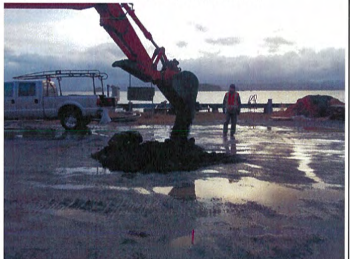
Photo 4. Advancing Test Pit TP9 (facing southwest)
