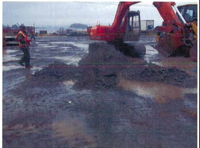
Photo 2. Advancing Test Pit TP13 (facing southwest)
