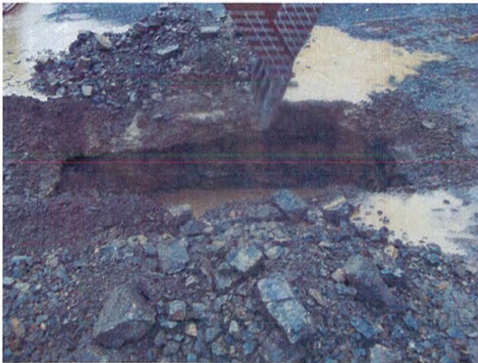
Photo 1. Advancing Test Pits .
