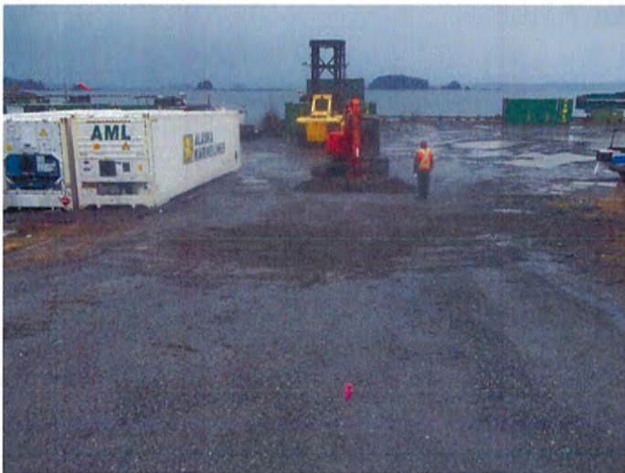
Photo 3. Advancing Test Pit TP6 (facing southwest)
