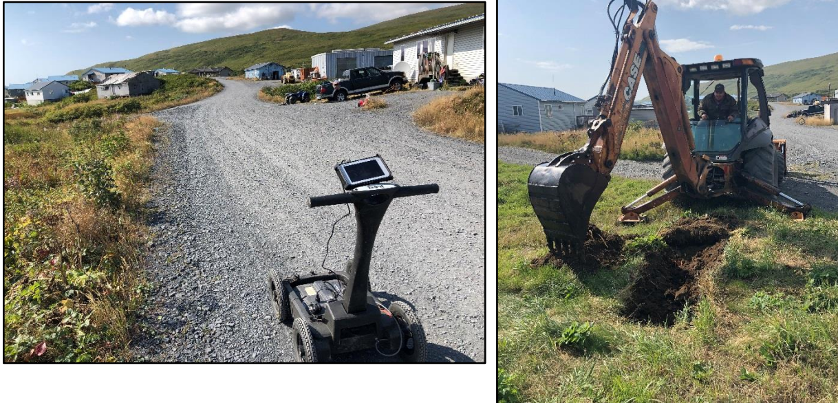
Image 1: GSSI UtilityScan 350 MHz HS GPR System (left) and Test Pit Excavation with Mayor Dan McCoy (right).
