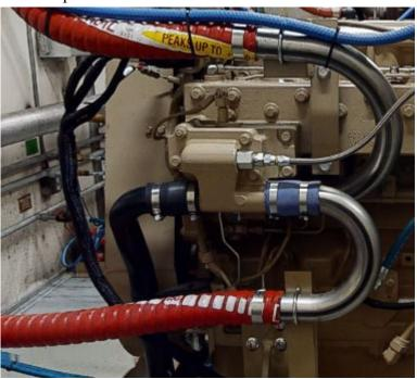
3. 6090HFM - Remove coolant tank and other accessories that are not required. Manifold vent lines into a single connection near the front with a 3/8" NPT quarter turn gauge cock isolation valve.
