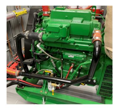
*Note that <u>Ruby Gen #3</u> 4045AFM MUST be provided with a steel tube to the front as shown.*
