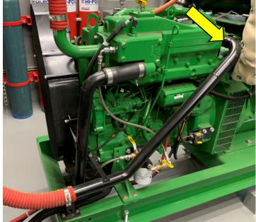
*Note that <u>Platinum Gen #1</u> 4045TFM will NOT be provided with a steel tube to the front as shown.*
